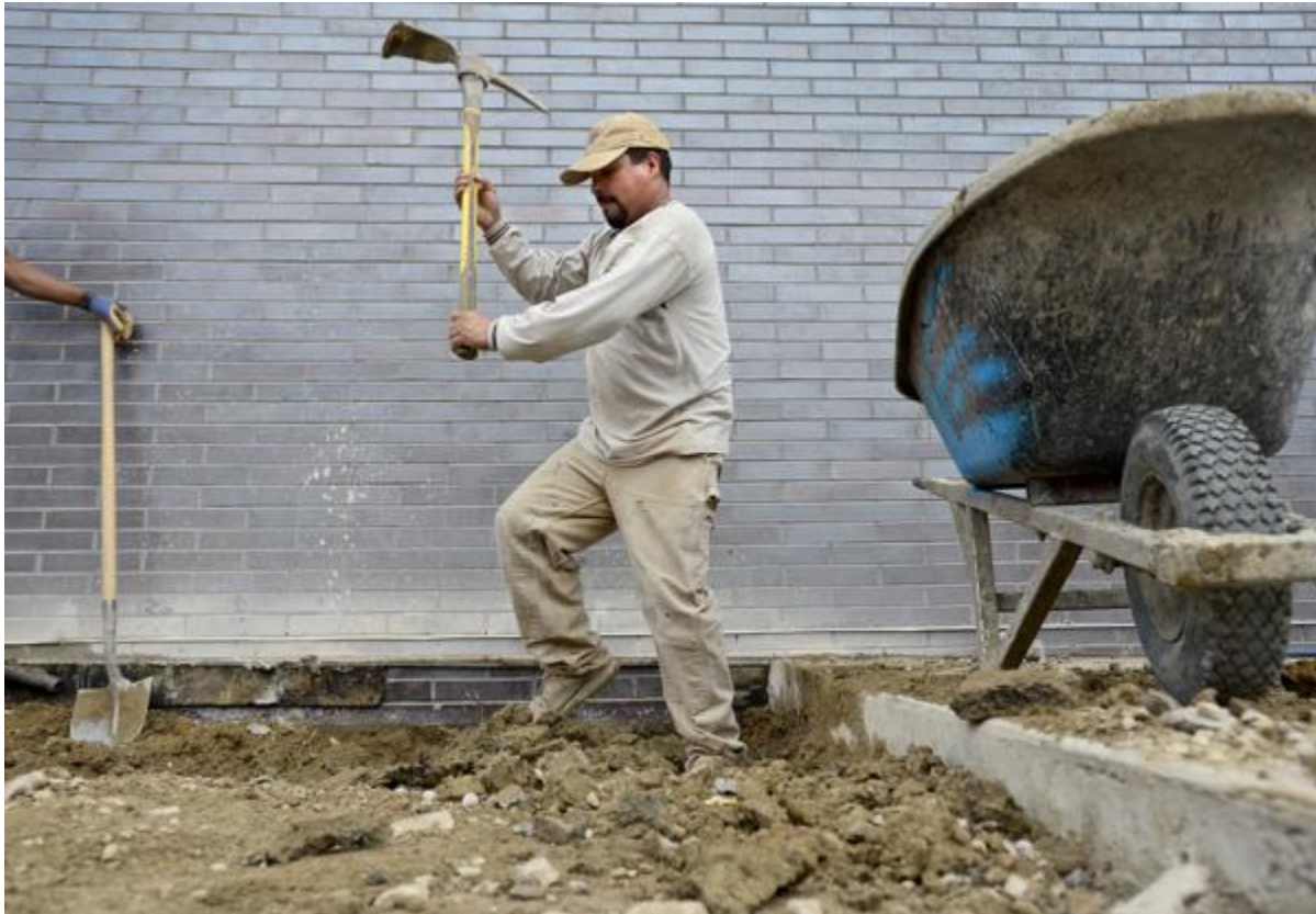
Antonio Alvarado of Total Concrete Services Inc. uses a pickaxe to break up the ground on Thursday in front of Roosevelt Park Apartments in Longmont. A statue depicting Teddy Roosevelt on the back of a train during his whistle stop tour in 1900 will be installed in late September. (Matthew Jonas / Longmont Times-Call)
